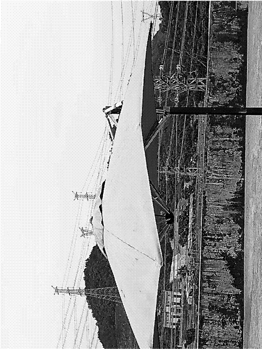
FIG. 10 (w/ flexible panel covering canopy frame assembly; the flexible panel covers on top of the long ribs including support arm)
